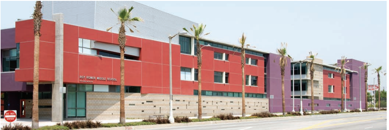
A view of LAUSD's Roy Romer Middle School project.
